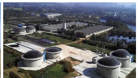
Ratchaburi Farms Biogas Project at SPM Farm
